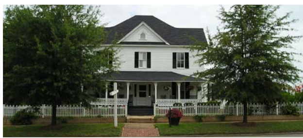
(a) Traditional two story wooden building along a main thoroughfare in Greensboro as pictured at greensboroga.gov
