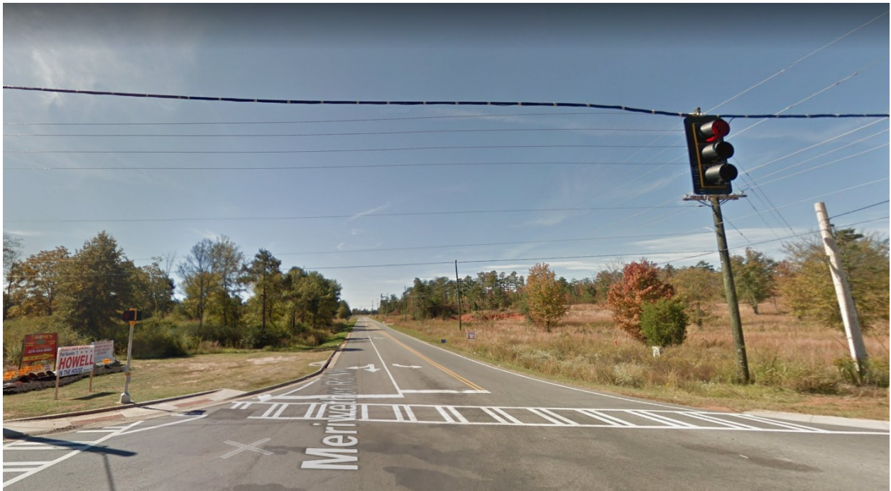
Photo taken from intersection facing west on Meriwether Rd, site is on the right
